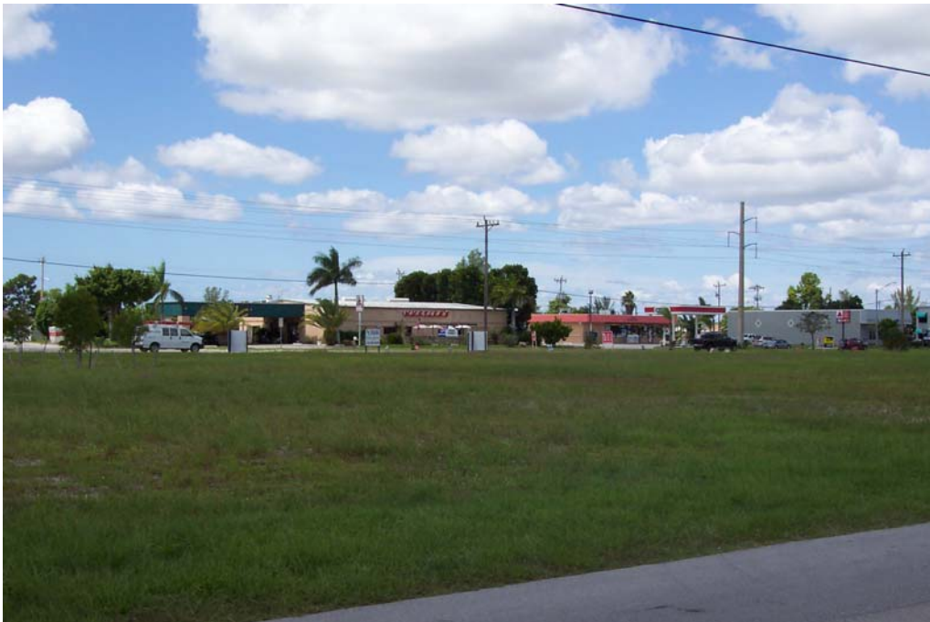
NW'LY VIEW OF THE SUBJECT SITE, AS SEEN FROM SE SANTA BARBARA PLACE
