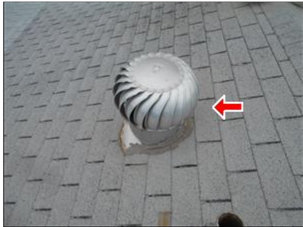
9.2 Picture 2 Turbine vents
