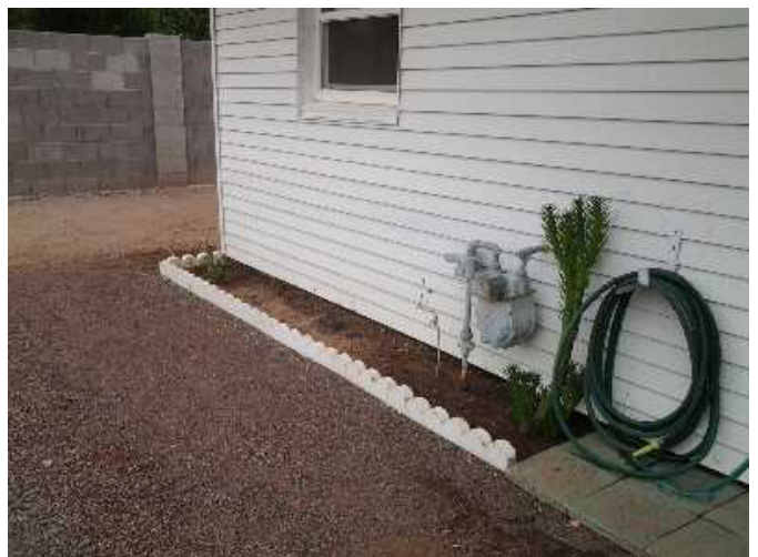
exterior covered by vinyl siding
