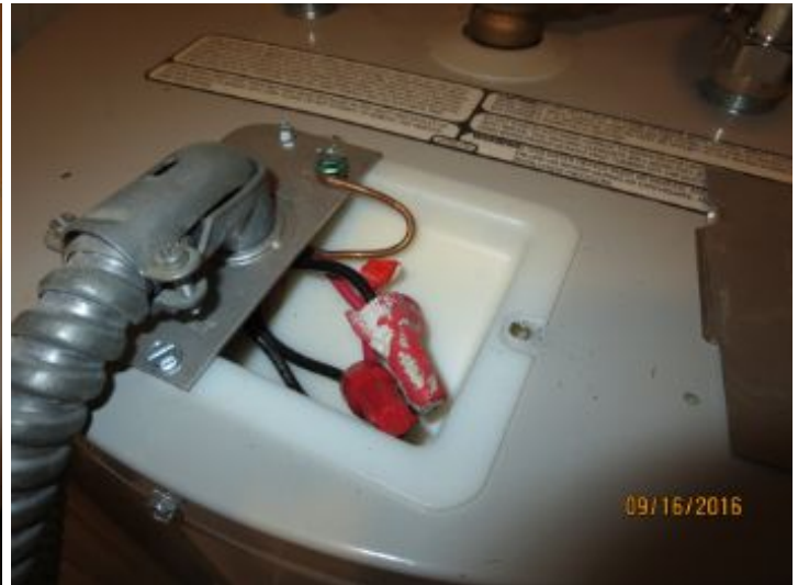
The electrical connection appears to be functional at time of inspection
