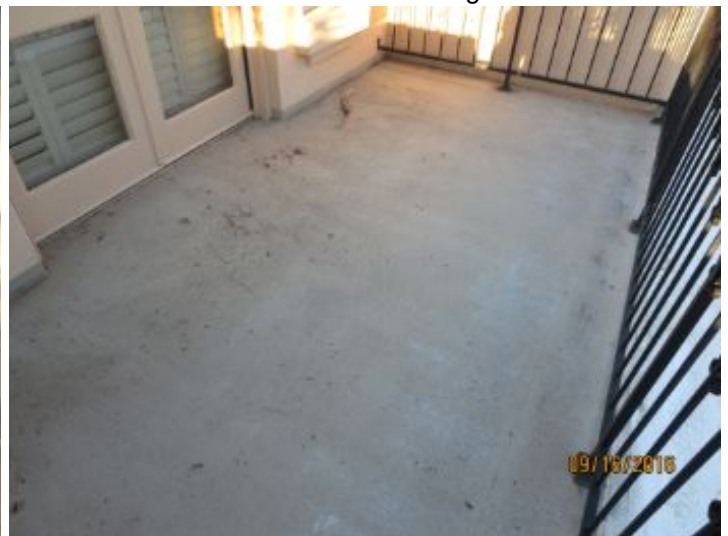
Northeast bedroom deck view
