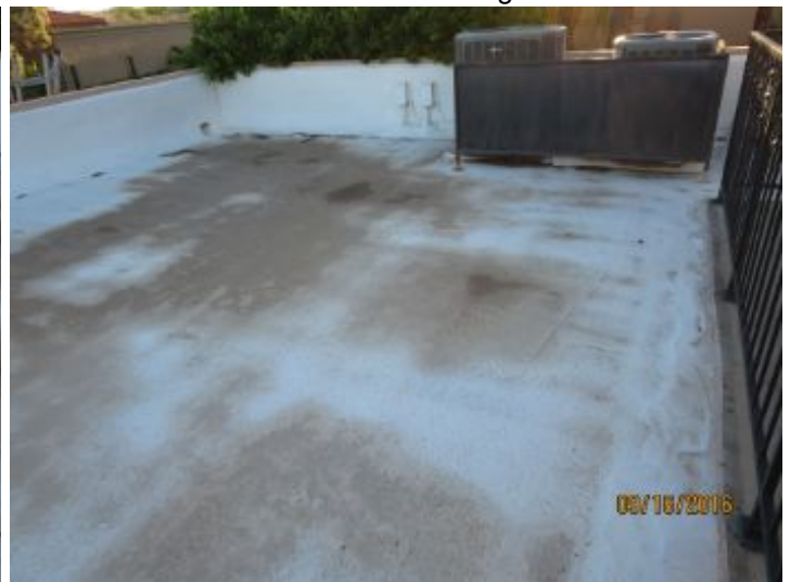
Lower Roof view looking east
