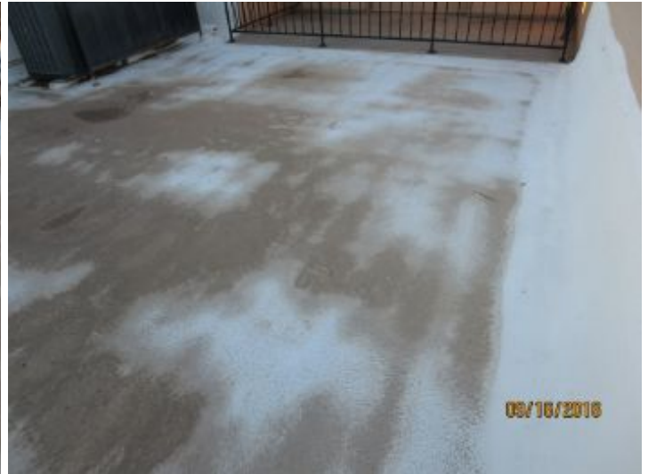
Lower Roof view looking south
