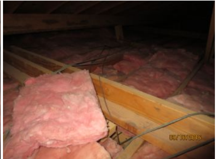
Fiberglass batt insulation installed between roof trusses.
