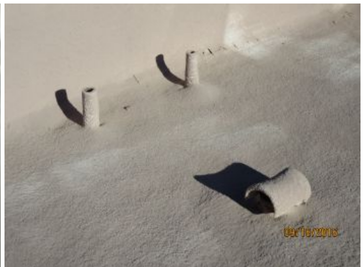
Vent caps appear functional
