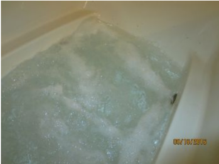
Whirlpool tub operated at time of inspection
