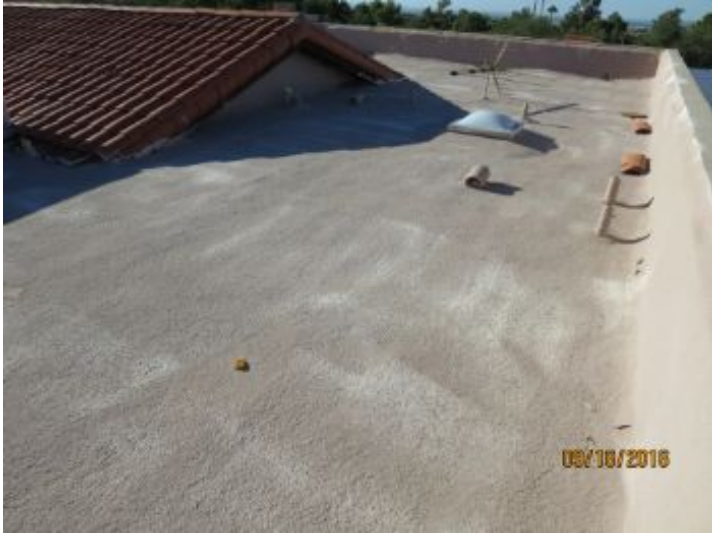
Roof view looking south
