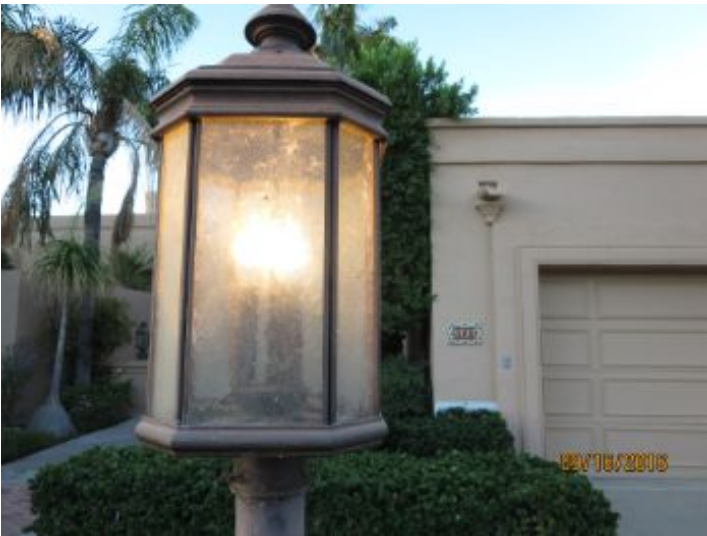
Exterior lighting was operational at time of inspection.
