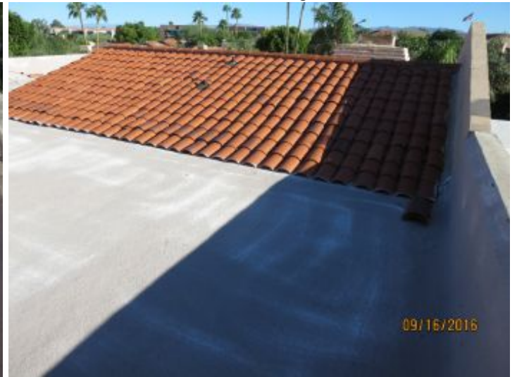
Roof view looking north
