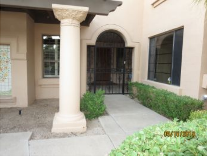
Front entryway appeared to be in good condition at time of inspection.
