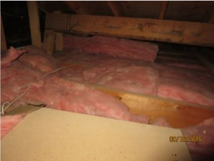
Fiberglass batt insulation installed between roof trusses.
