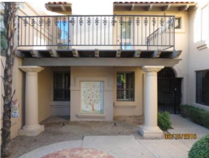
North side of house
