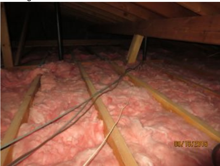
Fiberglass batt insulation installed between roof trusses.
