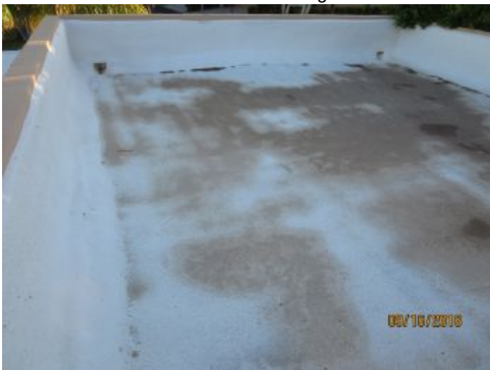
Lower Roof view looking north
