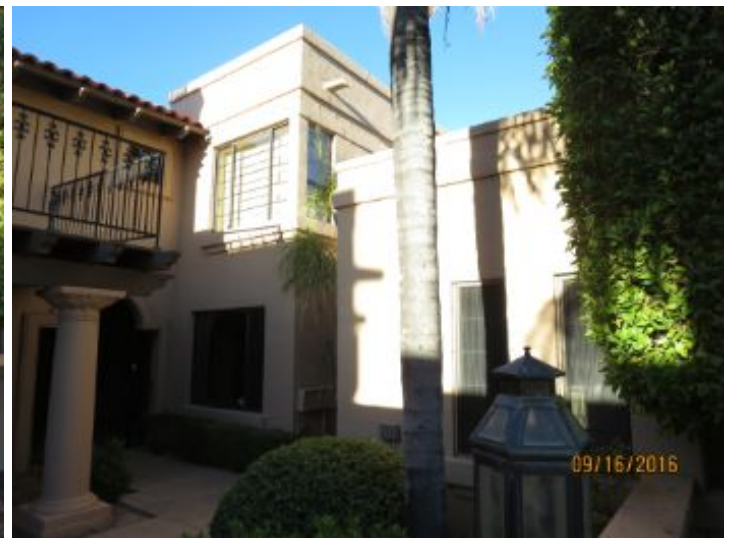
East side of house
