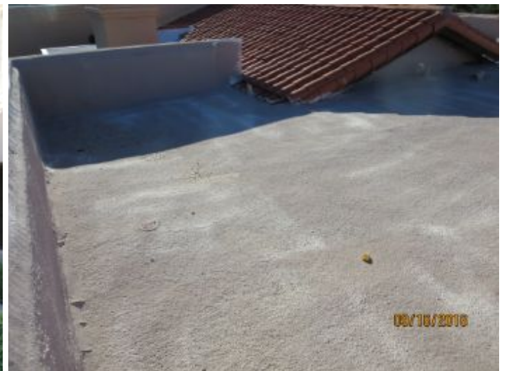
Roof view looking east
