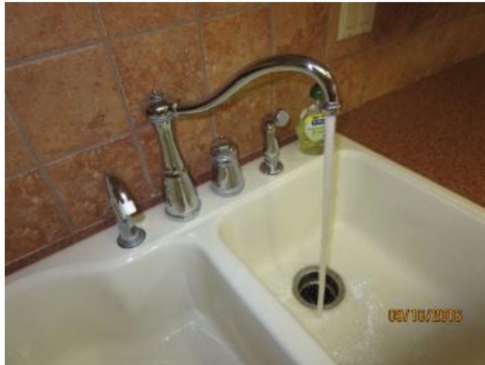
Kitchen faucet appeared functional at the time of inspection
