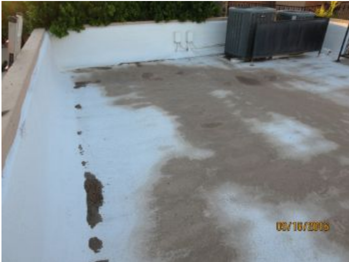
Lower Roof view looking east
