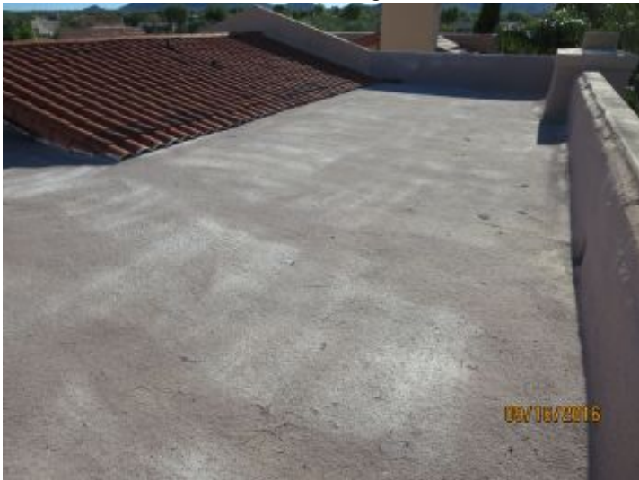
Roof view looking east
