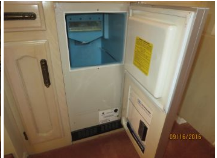
The ice maker at the wet bar was not turned on at the time of inspection - not tested.
