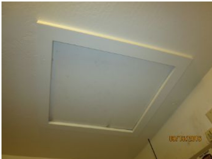
Location 1: 2nd floor northeast guest bedroom ceiling
