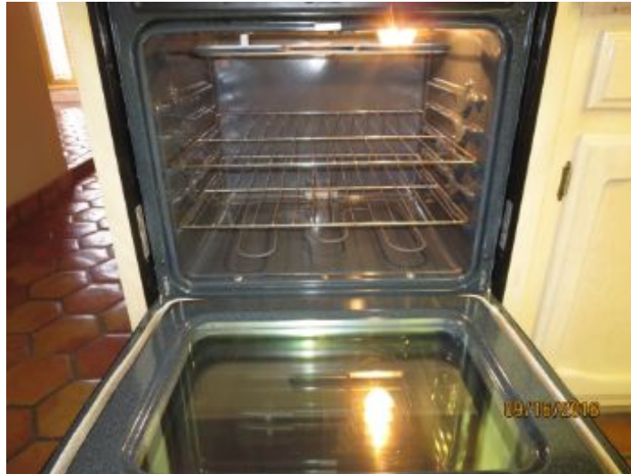
Oven element heated at time of inspection
