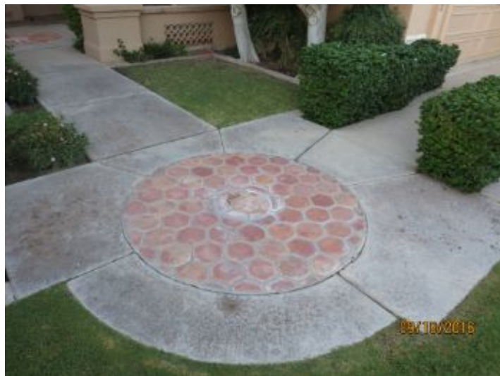
Concrete/tile sidewalks appear to be in good condition with common cracks noted.
