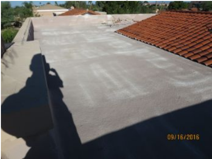
Roof view looking west
