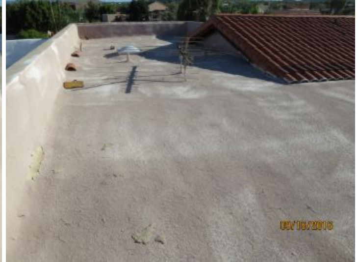
Roof view looking north
