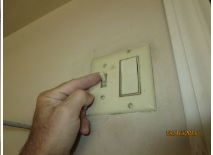
Garage door operates with wall switch.
