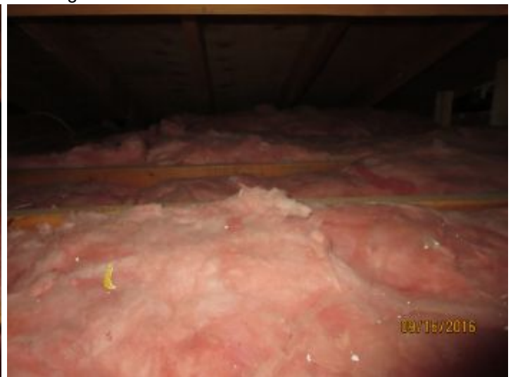
Fiberglass batt insulation installed between roof trusses.
