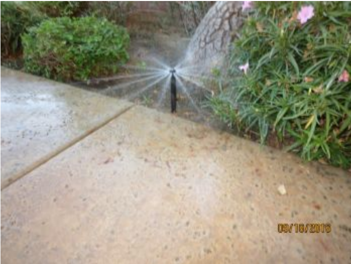
Recommend repositioning sprinkler/drip heads so they do not spray on front sidewalk.
